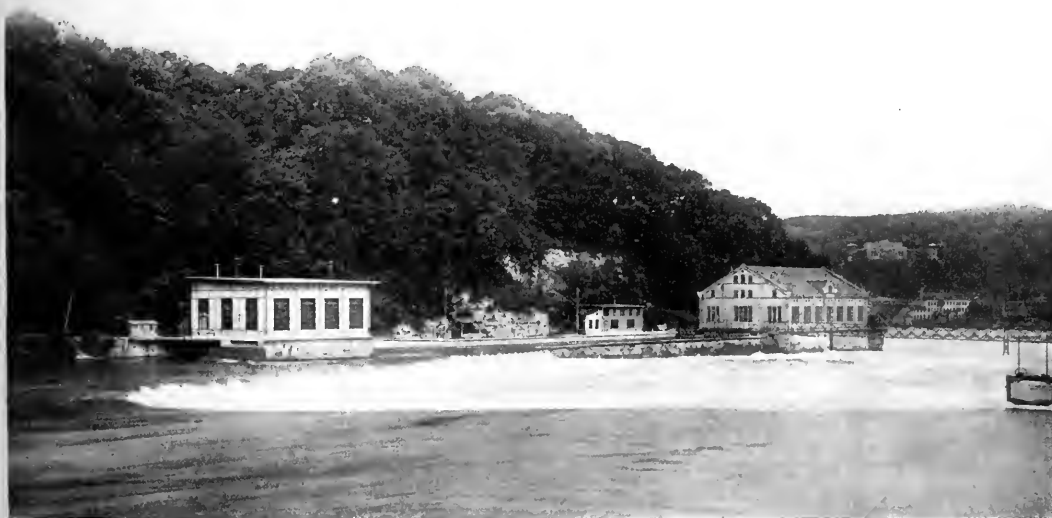
FIG. 1.—GENERAL VIEW OF BOTH POWER HOUSES, ON THE RHINE AT SCHAFFHAUSEN.
